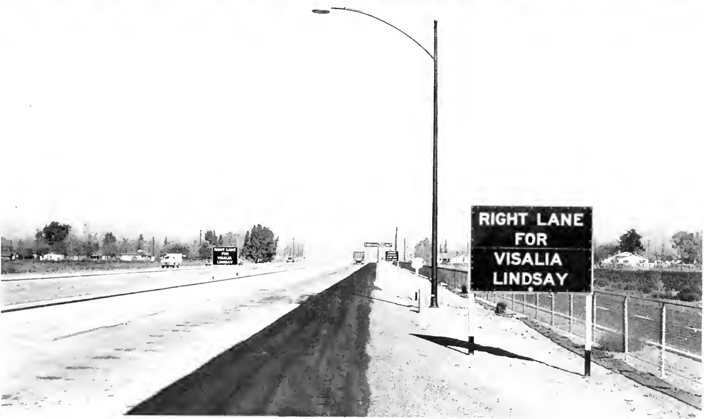
UPPER—Looking north from south end of Tulare By-pass. Overcrossing at left leads to business section of Tulare. LOWER—Looking north toward intersection of US 99 with State Sign Route 63, leading to Visalia and Lindsay.
